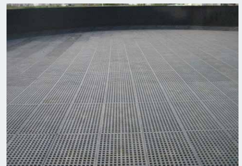
The stability of the structure after 48 hours at a load of 60 tonnes/m 2 (12,289 lbs/ft 2 ).
