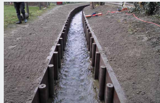
Bank reinforcement
